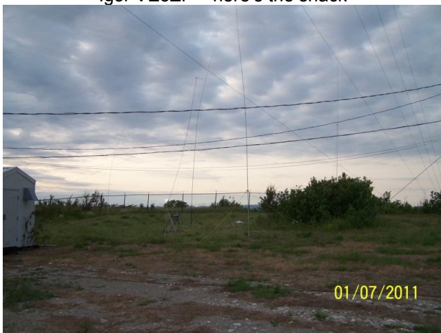
Phased verticals on 40 and 80 antennas
